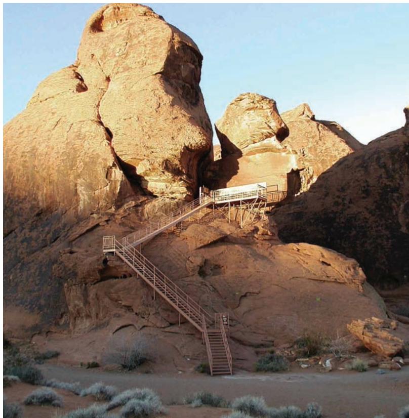
FIGURE 7.4—Viewing structure, Atlatl Rock, Valley of Fire State Park, Nevada. This kind of elaborate structure, designed to enable viewing while constraining climbing on and touching the rock and petroglyphs, is rare in the western United States.
